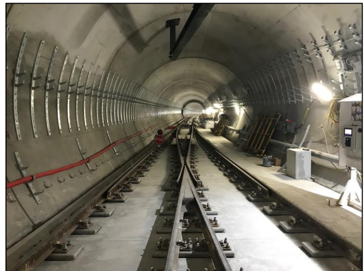
Looking back into the 'eastbound' platform (Above) and the eastbound tunnel (Below), showing the extra space to the right for an emergency walkway.
