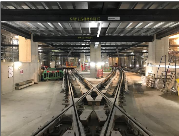
The track immediately beyond the 'eastbound' platform (Above) and the diamond crossover east of the station (Below).
