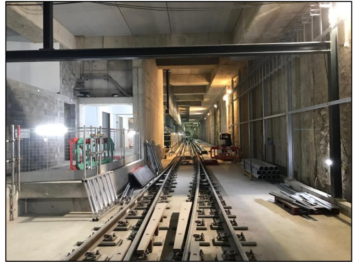
Looking back into the 'eastbound' platform (Above) and the eastbound tunnel (Below), showing the extra space to the right for an emergency walkway.
