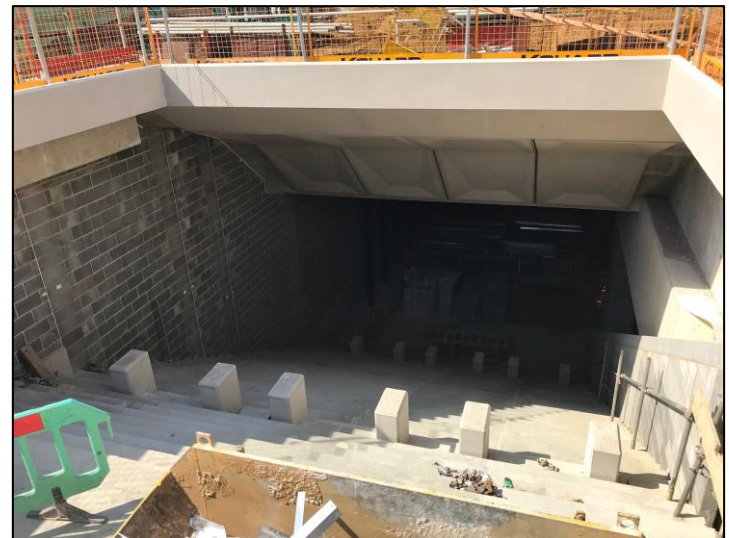
The escalator well. You can see where the cladding has been installed already above where the escalators will be.
